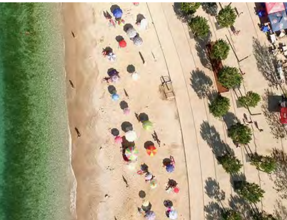
HIMARA WATERFRONT, 2014-16 Himara, Albania Client: City of Himara Architects: SON-group
