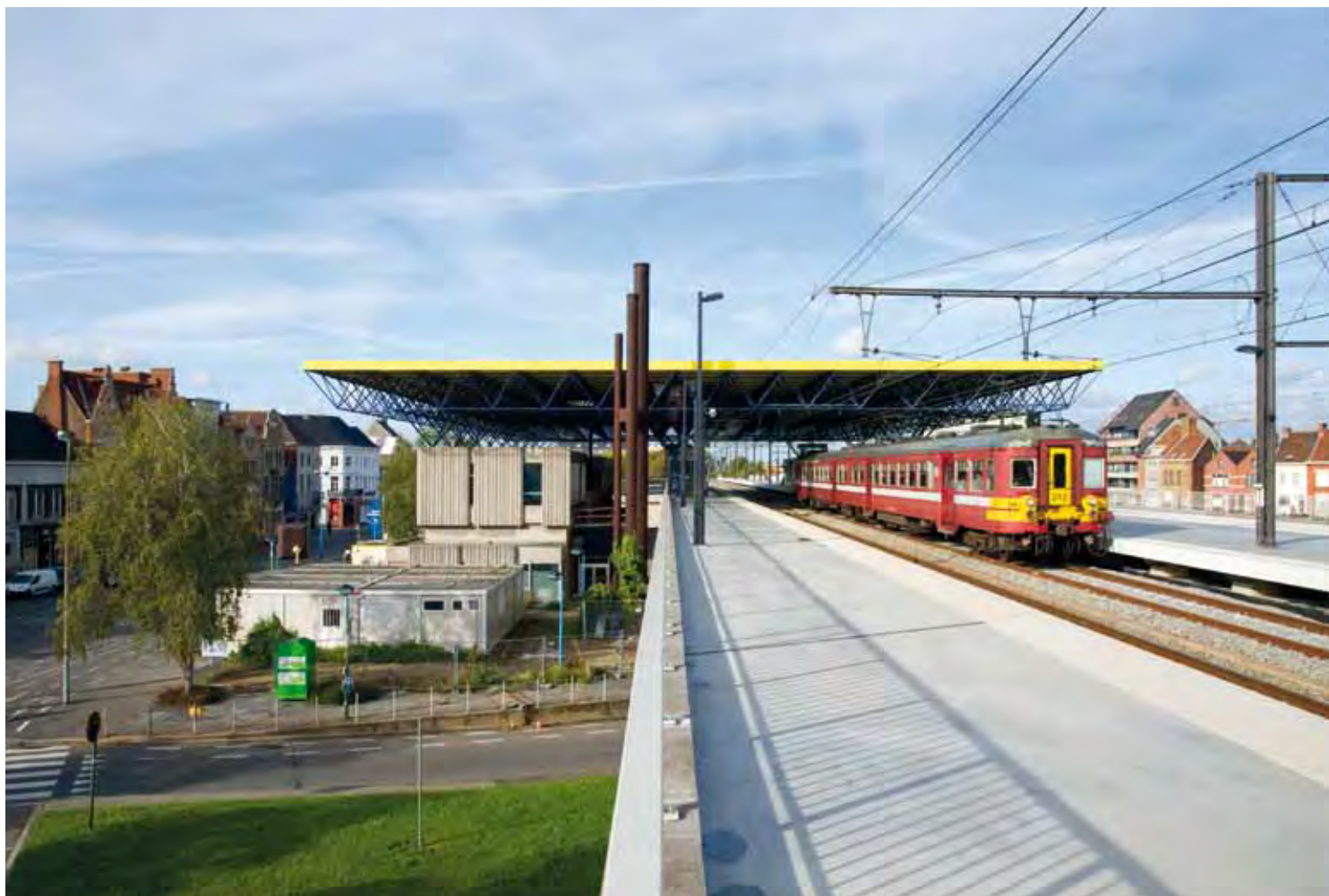
— The railway currently forms a barrier between the city centre and the Krottegem district. The project for the area around the station is partly focused on reinforcing the relationship between city and suburb once more.
